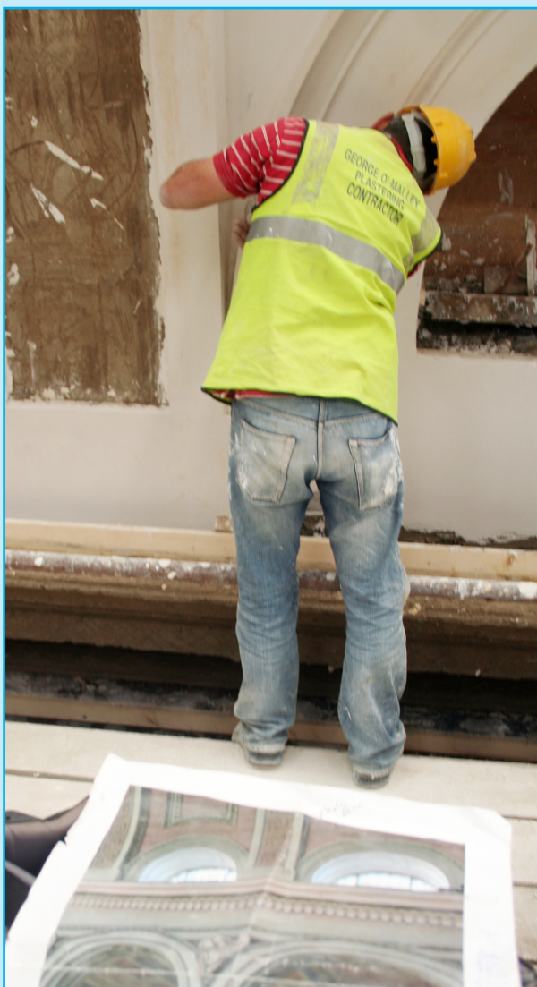
One of the professional plastering team at work at trial plasterwork in July.
