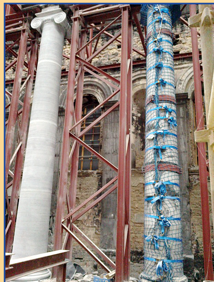
Picture shows the replica pillar in place alongside fire damaged pillar.
