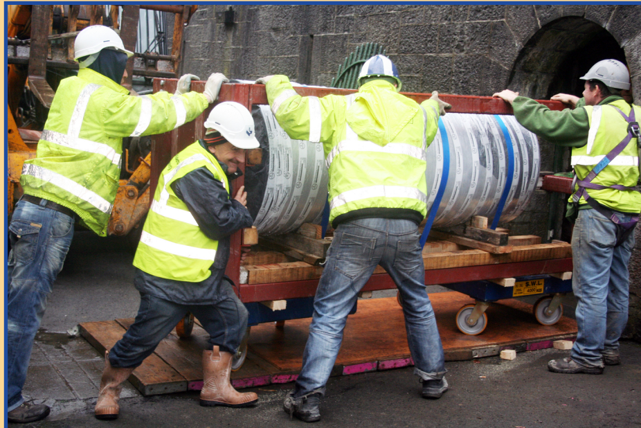
The replacement pillar is wheeled into the Crypt of the Cathedral manually.
