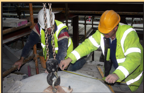
Pillar foundation stone being measured as workmen begin the process of setting it in place.
